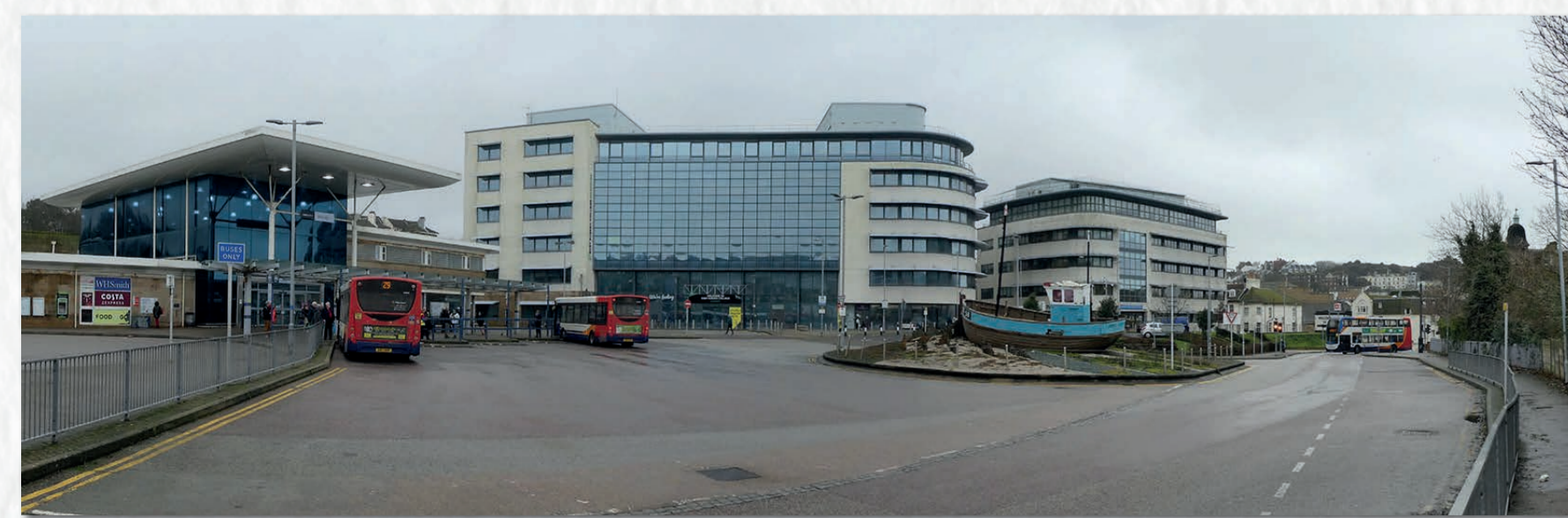
v1 - Station Plaza
