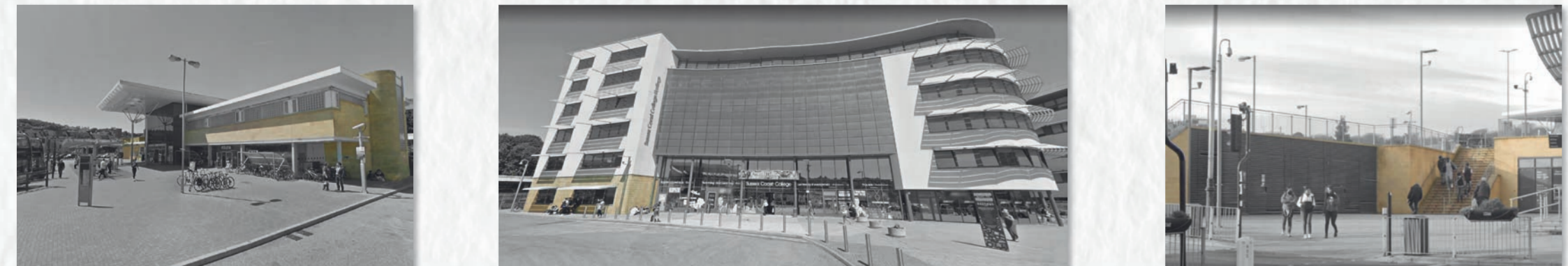
v1,v2,v3 - While most of the frontages on the plaza are render or render-like cladding there are splashes of sandstone dotted around. The station building has the most, alongside large areas of glass and white-painted metals
