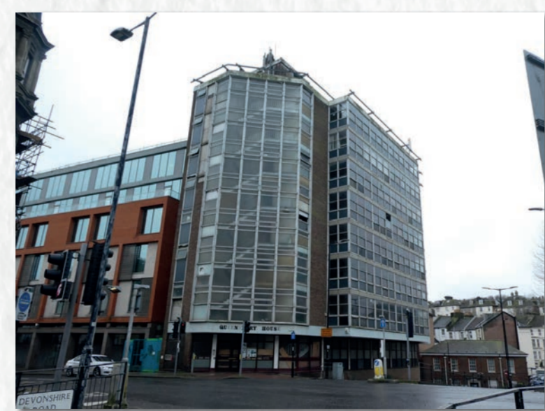
v2 - Queensbury House
