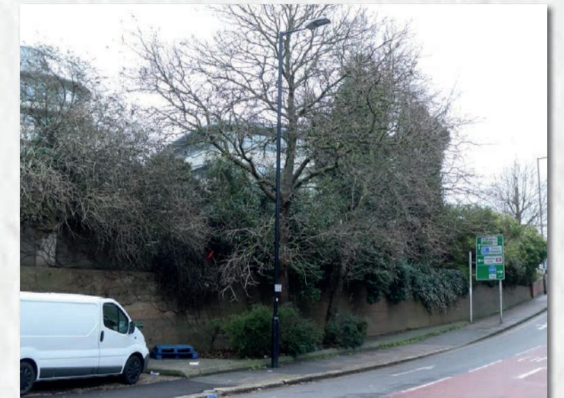
v2 - Retaining wall between Station Plaza and Priory St
