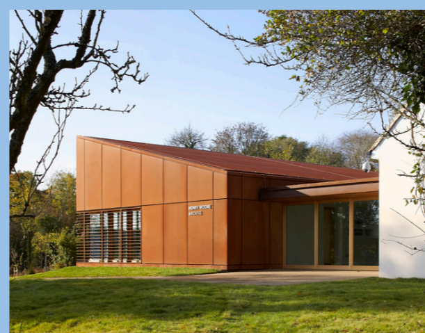
Henry Moore Extension HB Architects (London, 2017) Kingspan corten cladding
