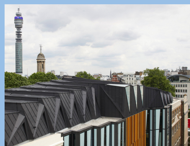
Which Headquarters Rooftop Extension Kohn Pedersen Fox Associates (London, 2018) Sweeping rolled-zinc roofing
