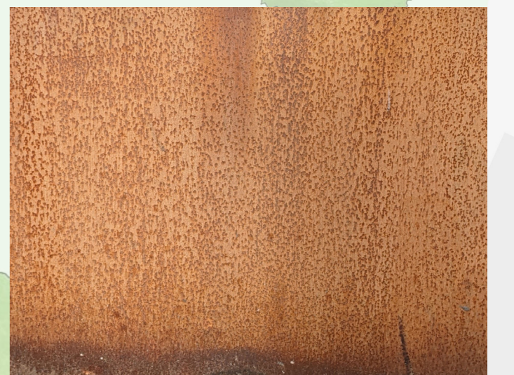
Corten steel is used throughout, celebrating the industrial heritage of the site and Norwich.
